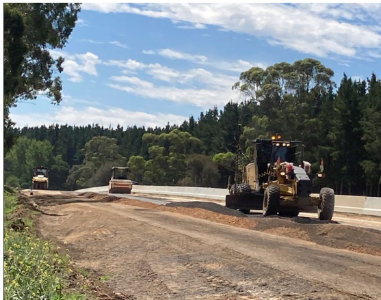
Princes Highway Corridor Upgrades Value: $ 80 m Construct Only (DIT)
