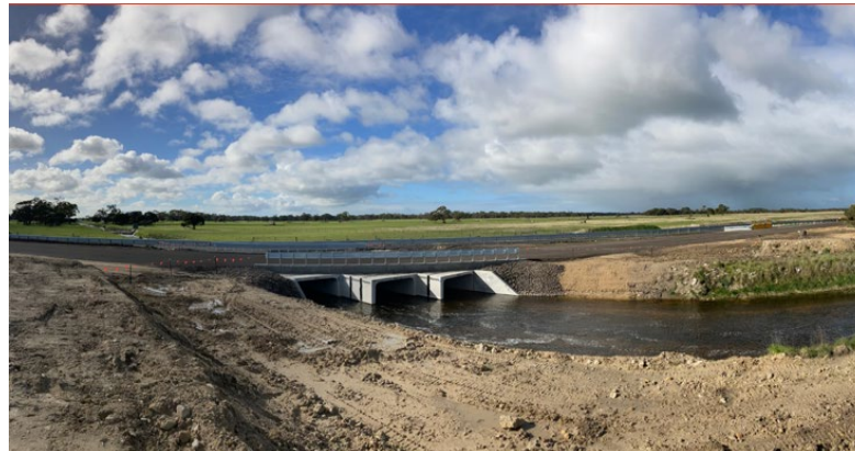
Various Bridge Replacements Value: $ 40m D&C Contract (DIT)
