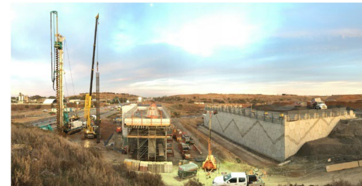
Piling works for the bridge over the Port River Expressway – June 2018
