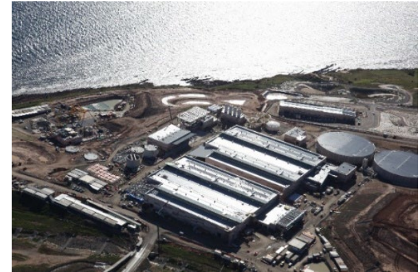
Adelaide Desalination Plant Value: $ 1.2 bn DBOM contract type
