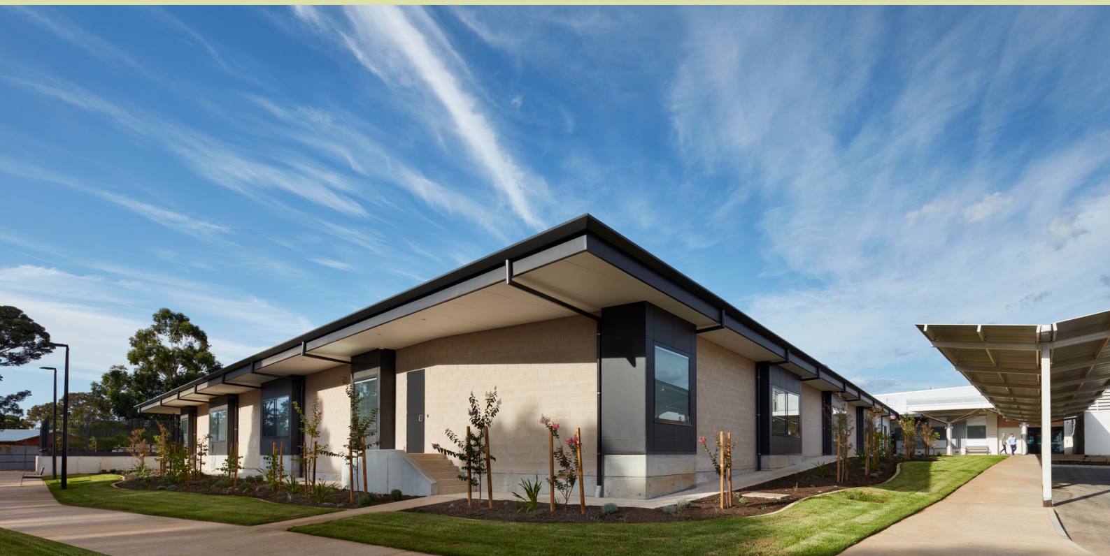
Photo supplied by Lendlease: Phase 2 of Repat Health Precinct Reactivation
