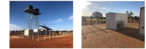
Example compound in Watinuma
